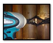
All you do is screw through the hard wood rail and into whatever you are fixing to, making sure that the bamboo panel is lifted off the ground 20-30mm. This avoids moisture absorbing.
